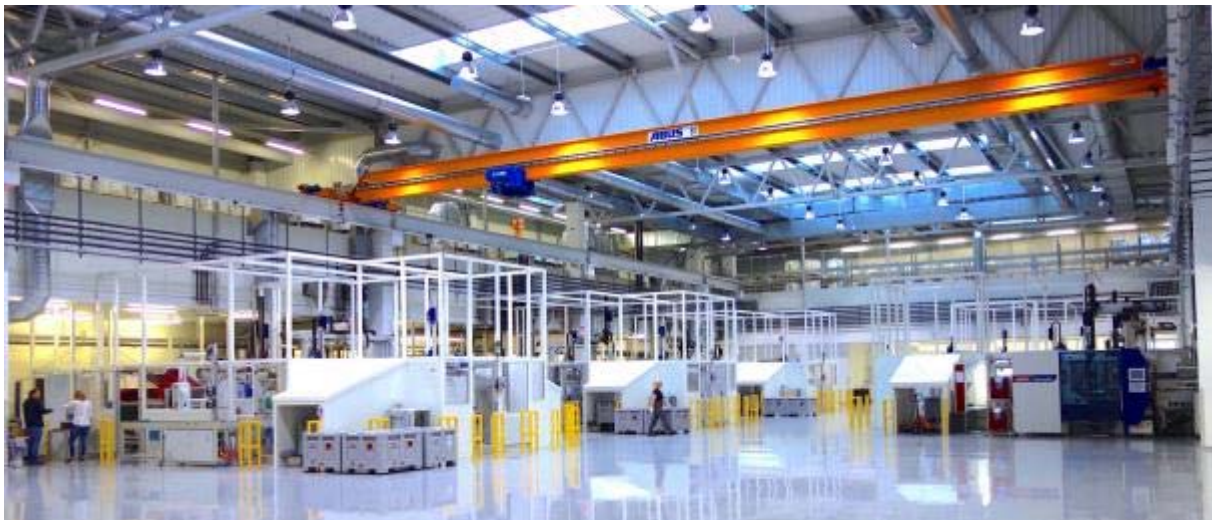
Fig. 2: The production plant of Buzek Plastic Poland in Plonsk, which was built following the principle of data networking according to an Internet 4.0 concept.
