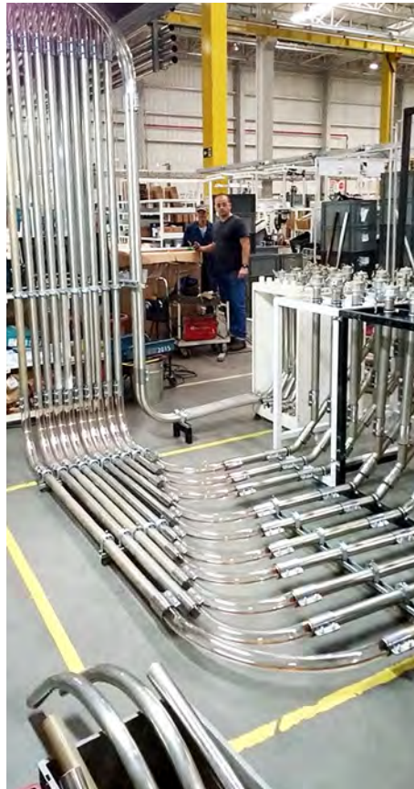
Conveying system detail after completion of the installation work.
