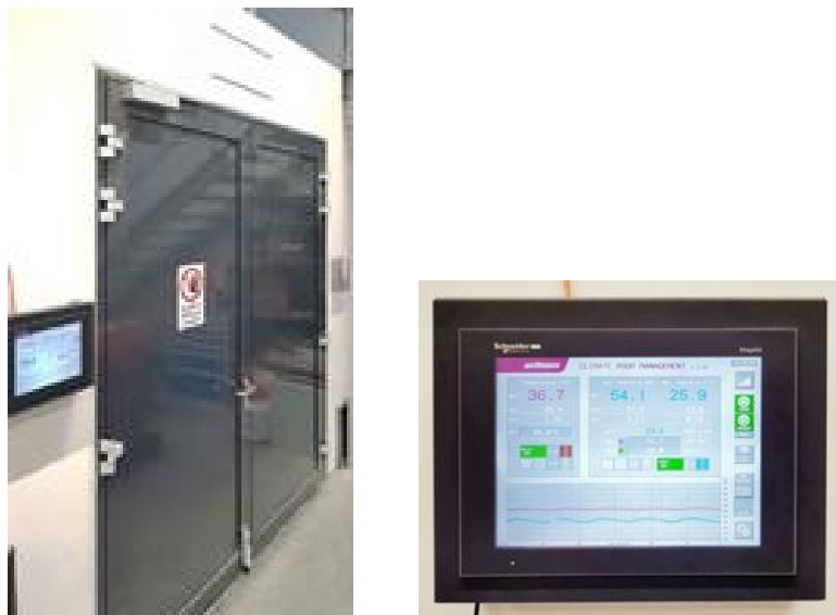
Hermetically sealed from the outside, the climatic conditions currently prevailing inside the chamber can be retrieved by using a touch terminal.
